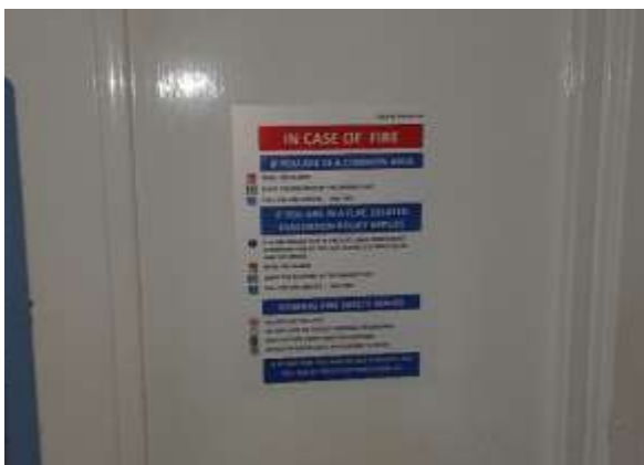
Figure 2: Worn and damaged paper notice replaced with a coloured laminated notice at The Martindales, Chorley
