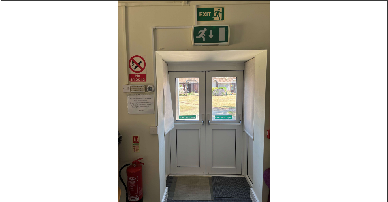
Photo No. 6 Community area Fire Exit.To the right Fire Routine notices All replaced with new signage.
