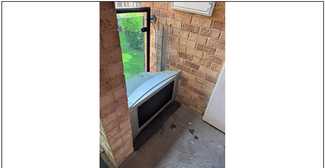
Photo No. 1 Personal items outside Flat 71
