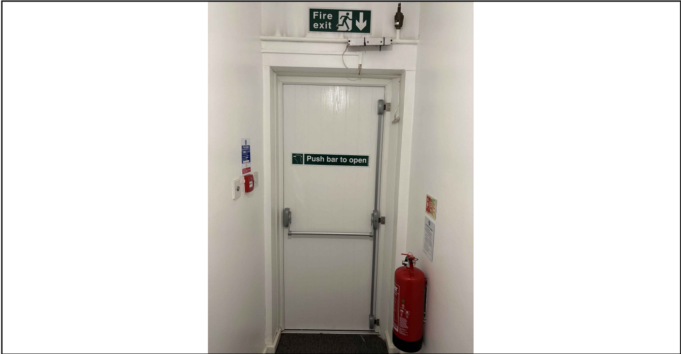
Photo No. 5 Fire exit from First floor
