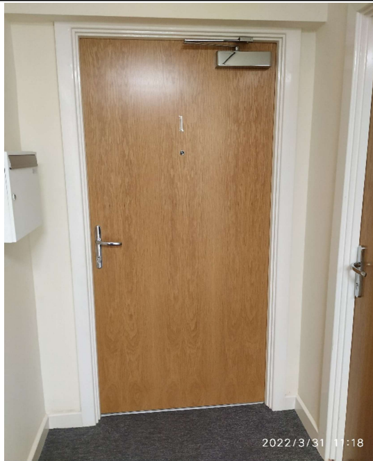
Flat Door construction, external letter box
