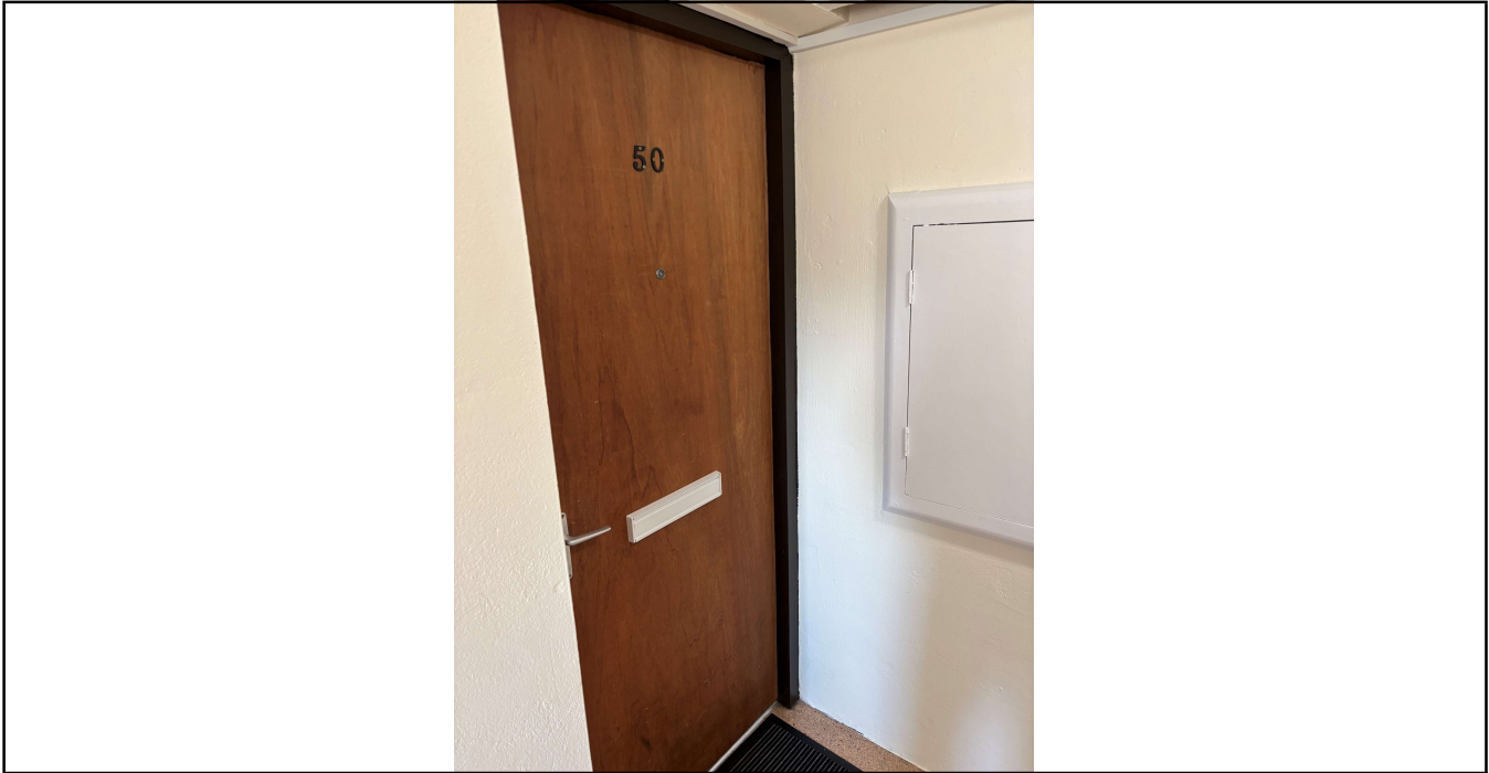
Photo No. 3 Standard Flat Door and utilities secure cupboard.
