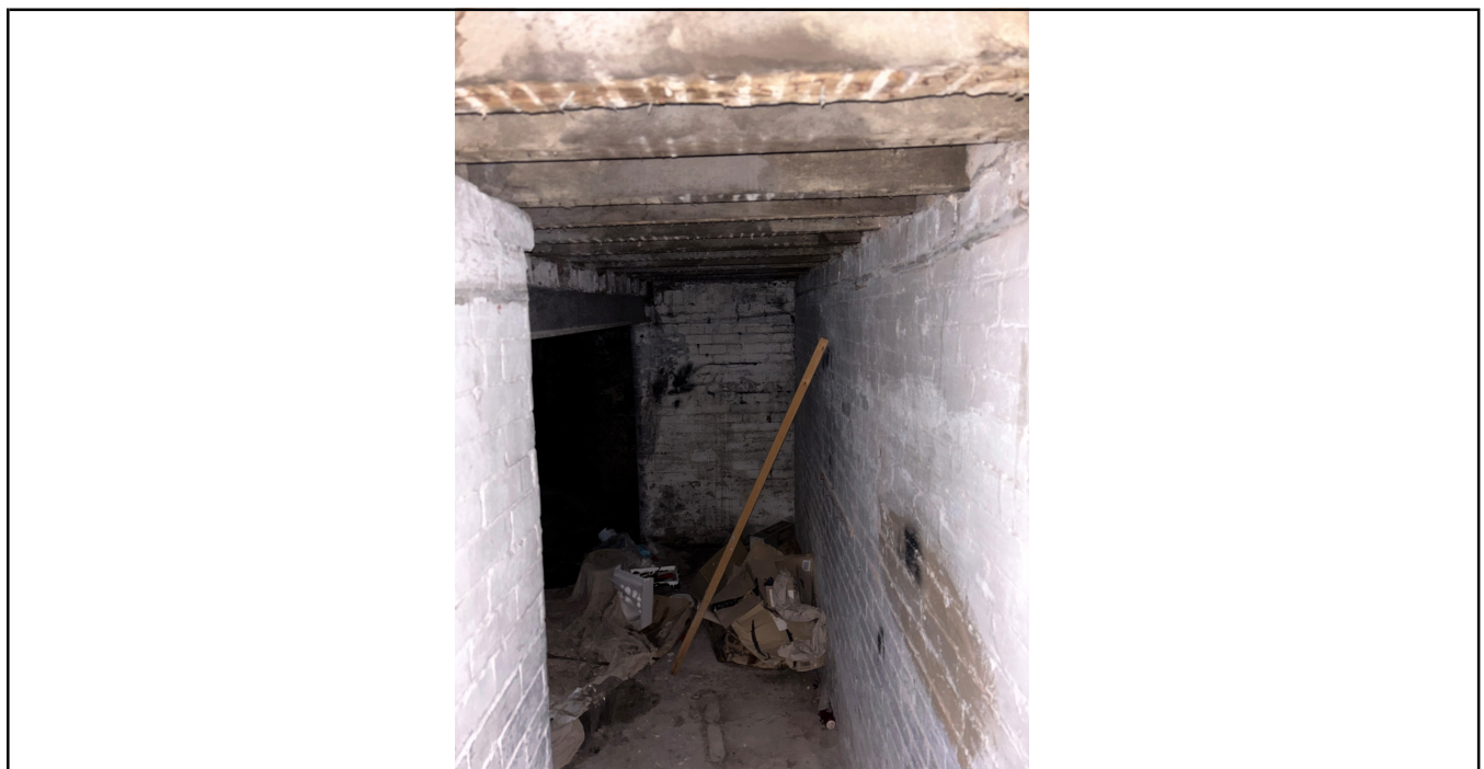
Photo No. 6 Fire separation in basement (picture from Flat 8)
