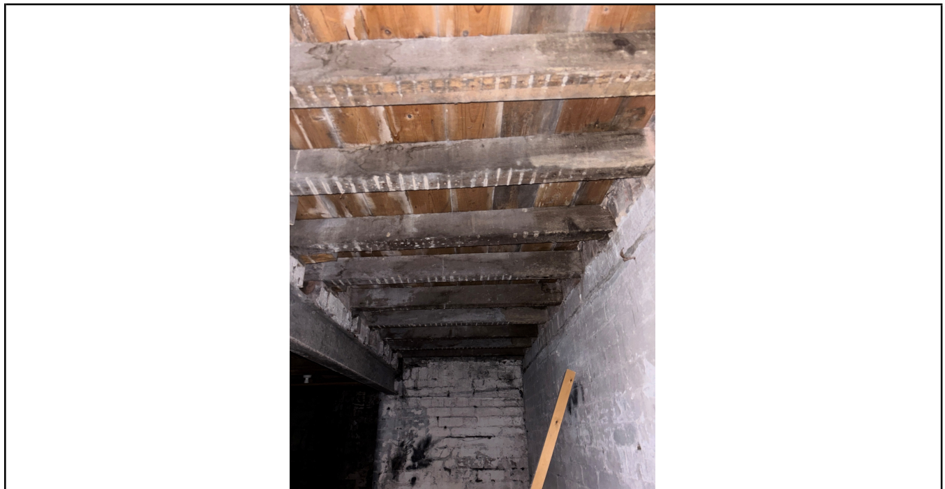
Photo No. 5 Fire separation in basement (picture from Flat 8)
