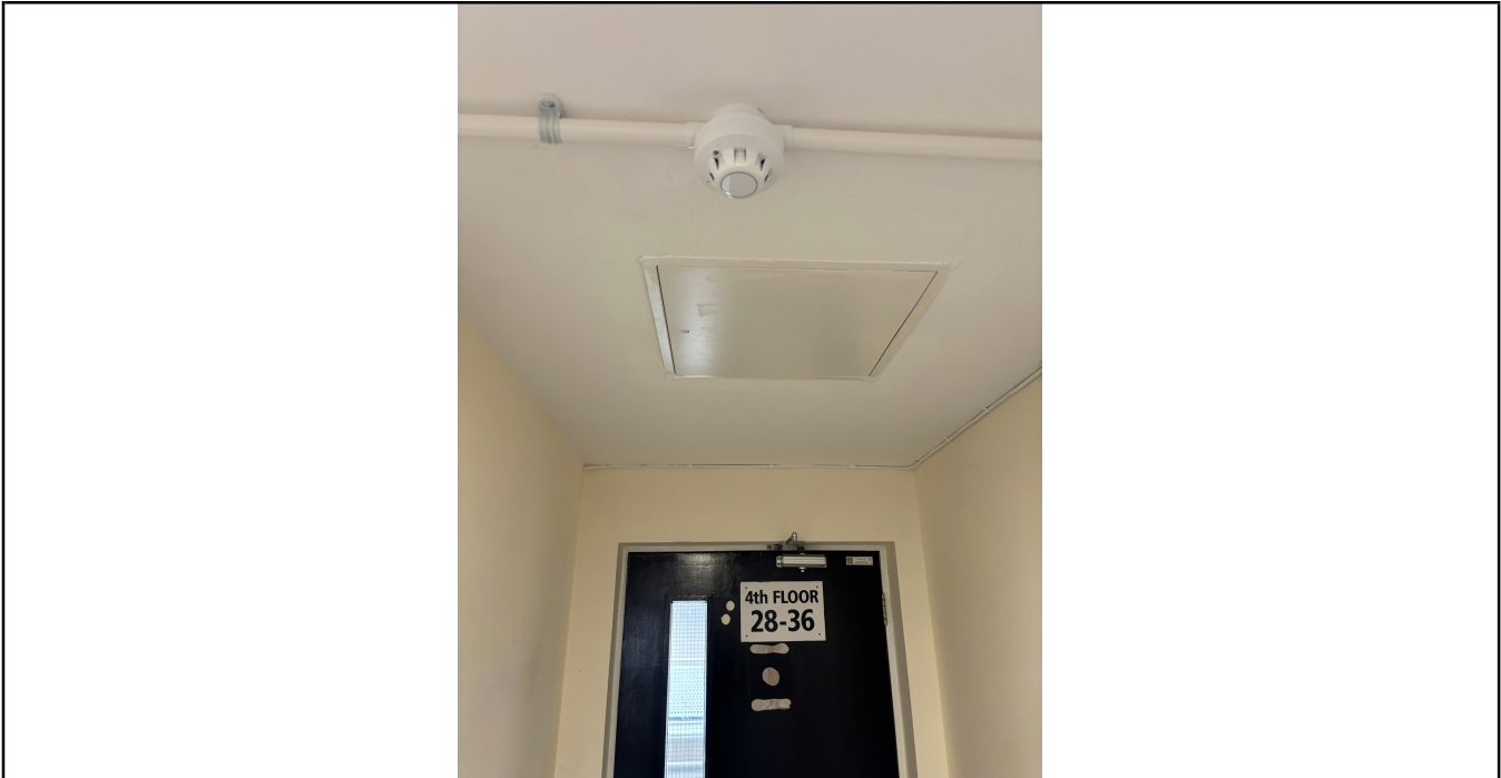
Photo No. 9 The loft hatch is of metal construction and complies to the latest standards
