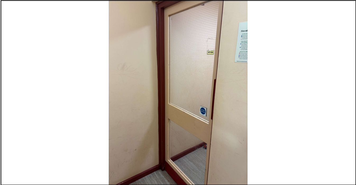
Photo No. 1 Lobby door protecting the stairs. Correct signage on the door.
