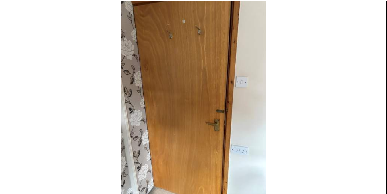
Photo No. 2 Ply flush internal doors fitted
