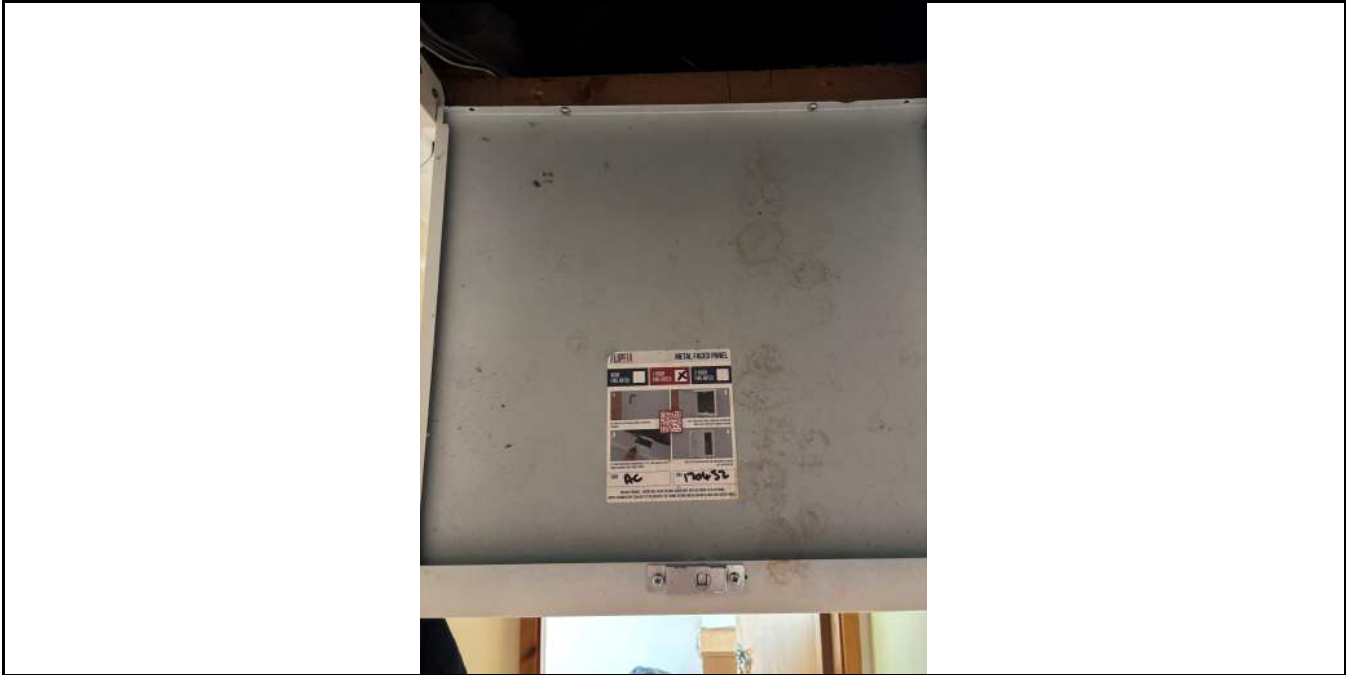
Photo No. 5 Loft hatch with appropriate fire resisting
