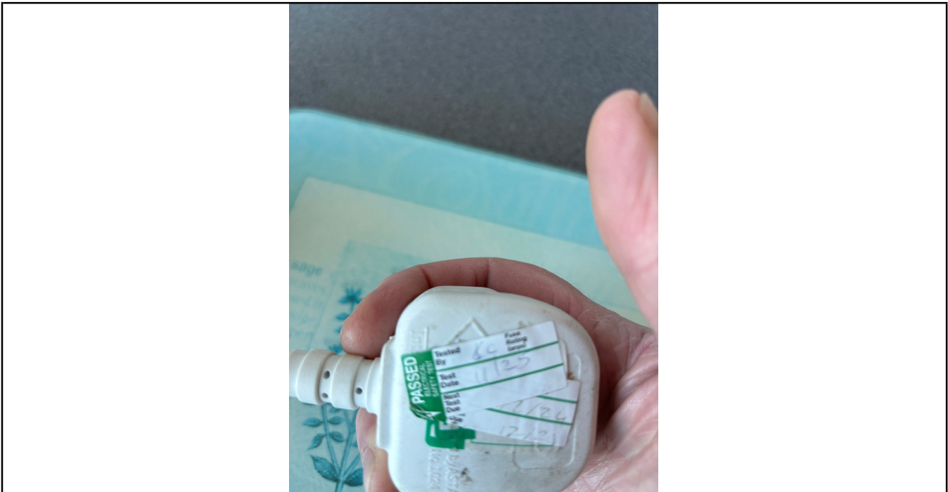
Photo No. 4 PA Testing. All items checked during the audit were in test date.
