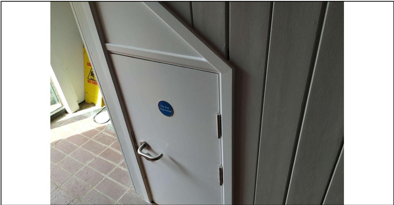
Photo No. 4 Fire Stopping Survey all staircase Fire Doors underneath access.
