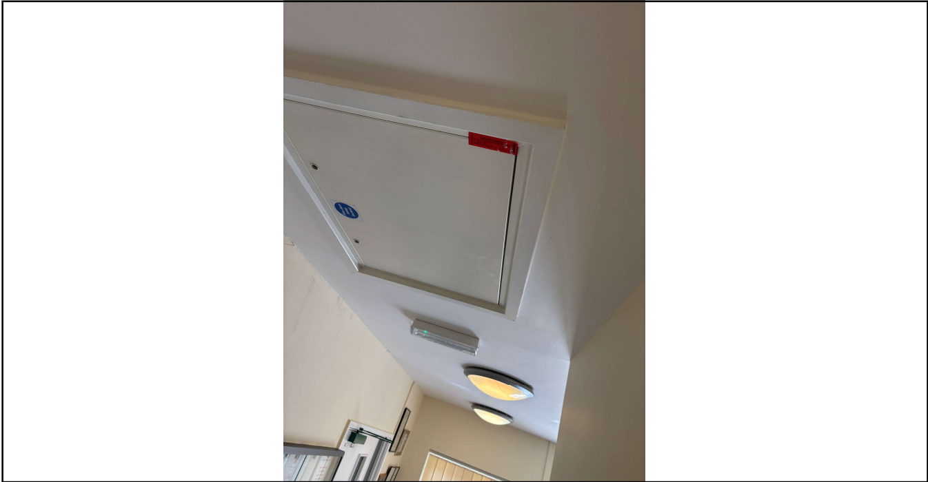
Photo No. 3 Community Building loft hatch, Fire stopping survey completed 2020 All office Doors and communal doors replaced.
