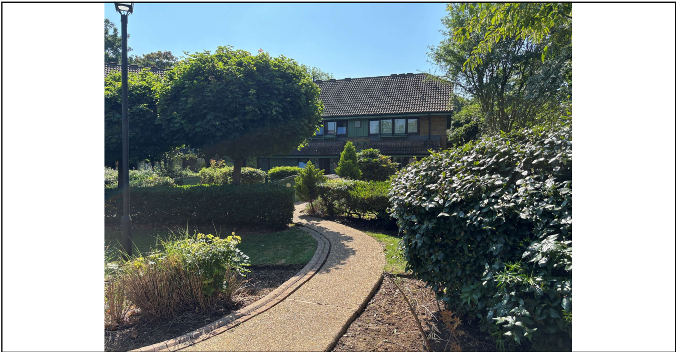
Photo No. 8 A well run scheme and well maintained.
