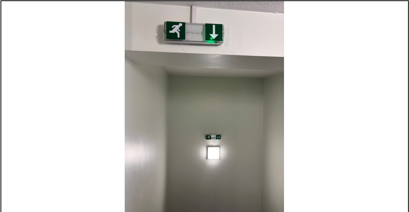
Photo No. 3 Satisfactory Signage throughout the block.
