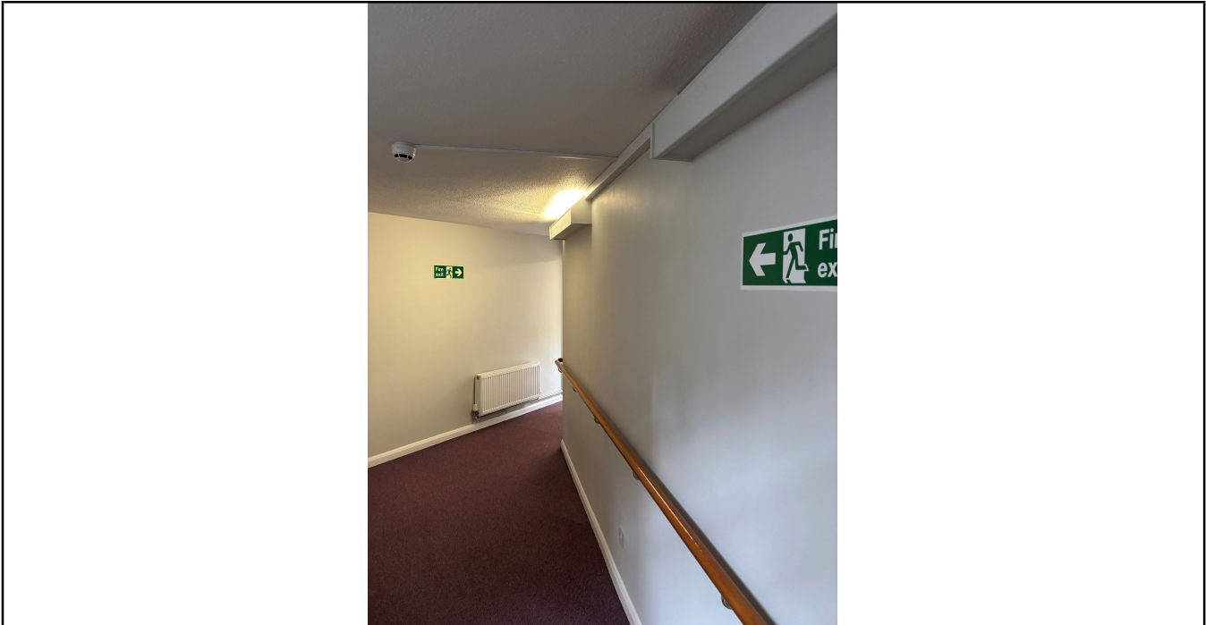
Photo No. 3 Correct signage throughout the building.
