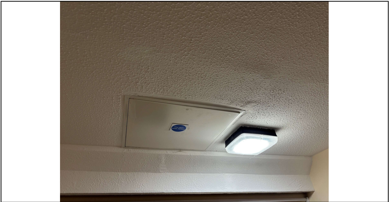
Photo No. 6 Fire Resisting Loft Hatch.
