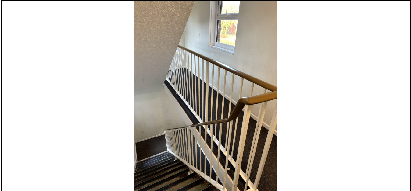
Photo No. 5 Escape route clear between 1st and ground floors
