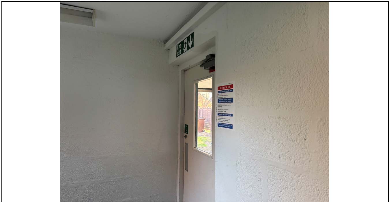
Photo No. 2 Main exit door
