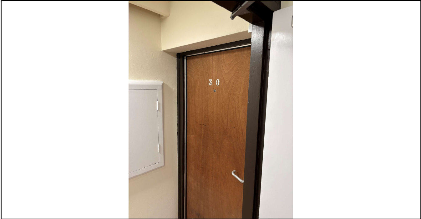
Photo No. 3 Standard Flat Door across the scheme.
