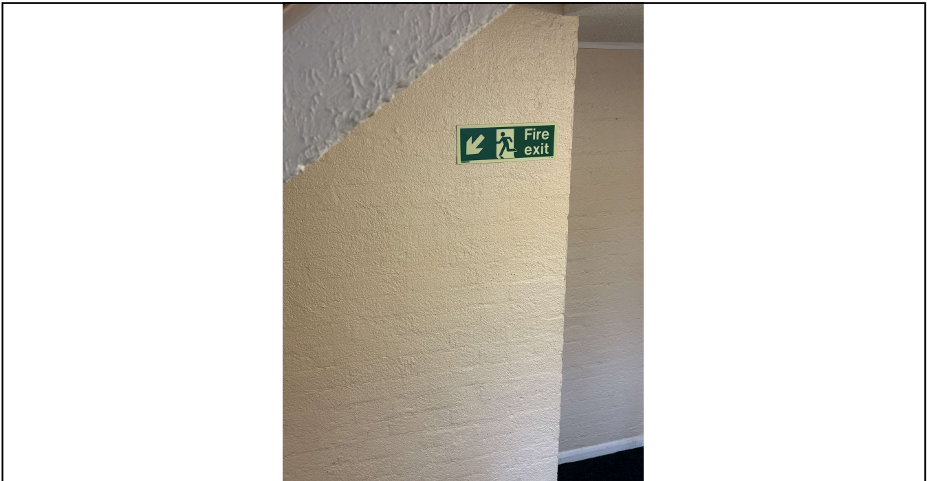
Photo No. 2 Exit Signage throughout the building
