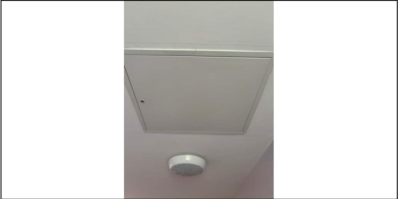
Photo No. 11 Typical loft hatch fitted
