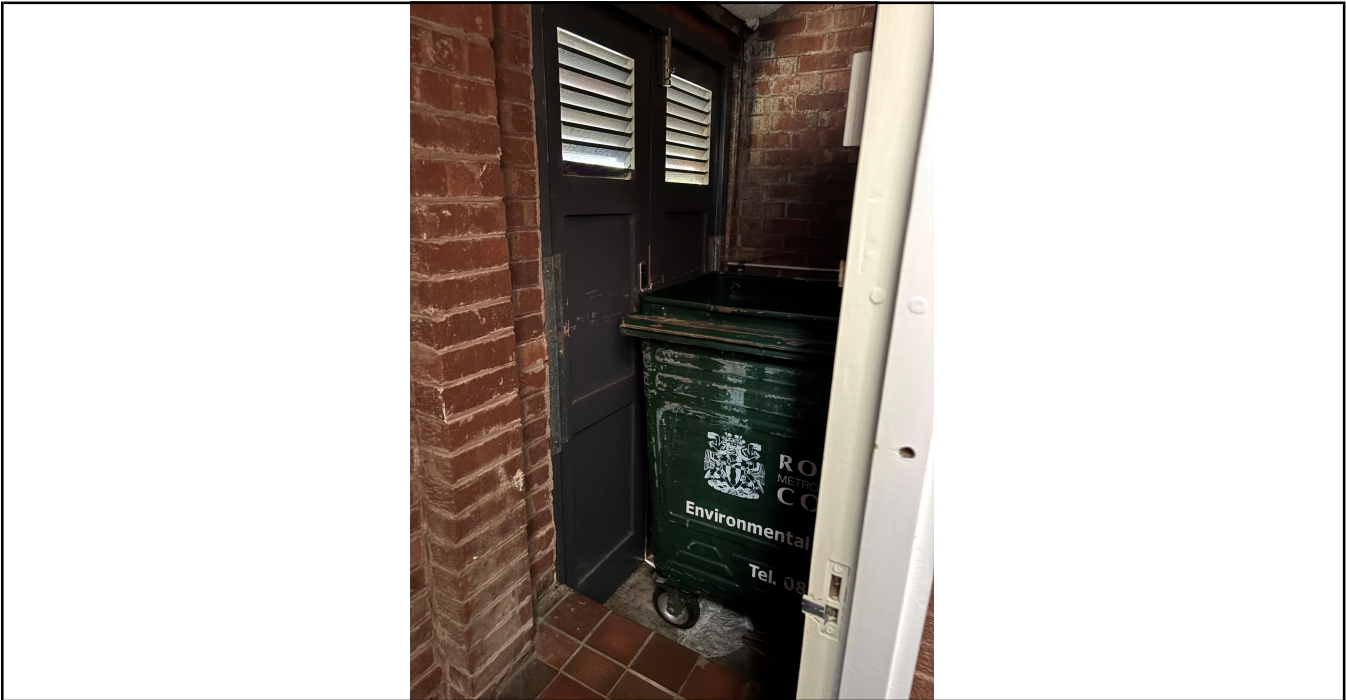
Photo No. 4 Bin store clean and tidy
