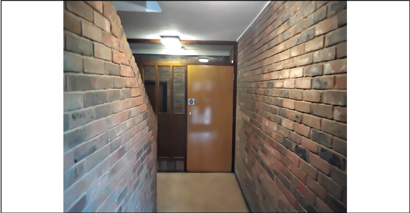
Photo No. 5 Communal first floor Smoke lobby.
