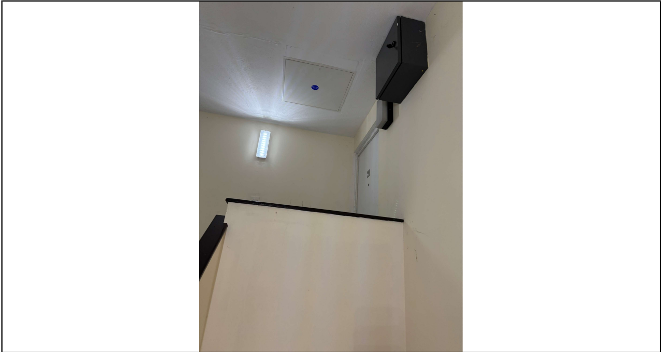
Photo No. 6 Fire Resisting Loft Hatch replaced from last FRA 2023.
