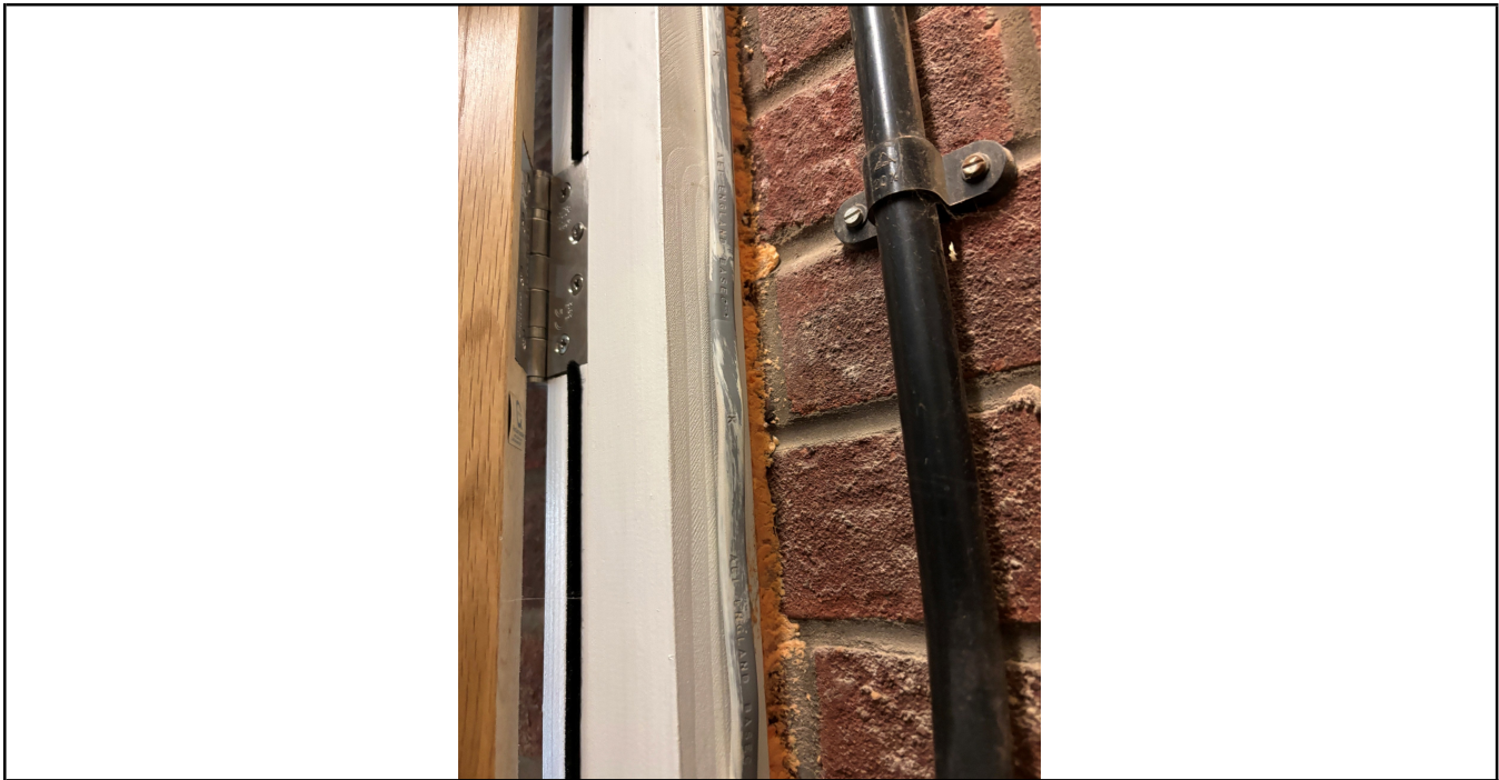
Photo No. 11 New door frames filled with pink foam
