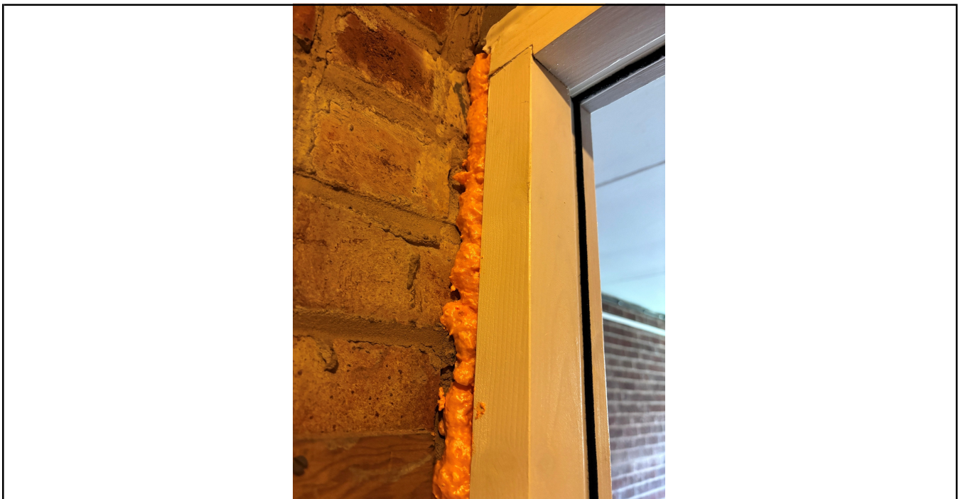
Photo No. 12 New door frames filled with pink foam
