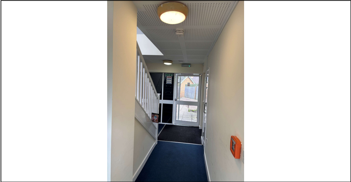
Photo No. 1 Access through main door into protected stairwell additional Rear Exit into communal garden area.
