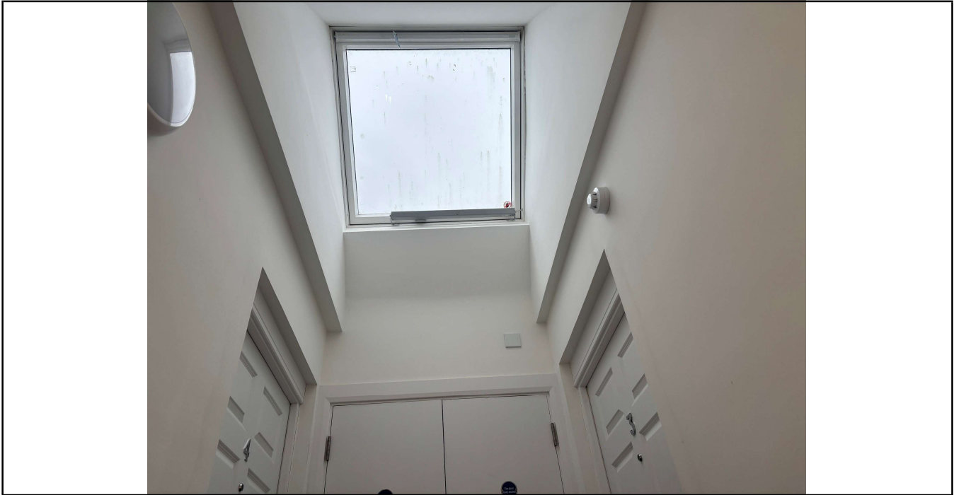
Photo No. 5 AOV and smoke detection.
