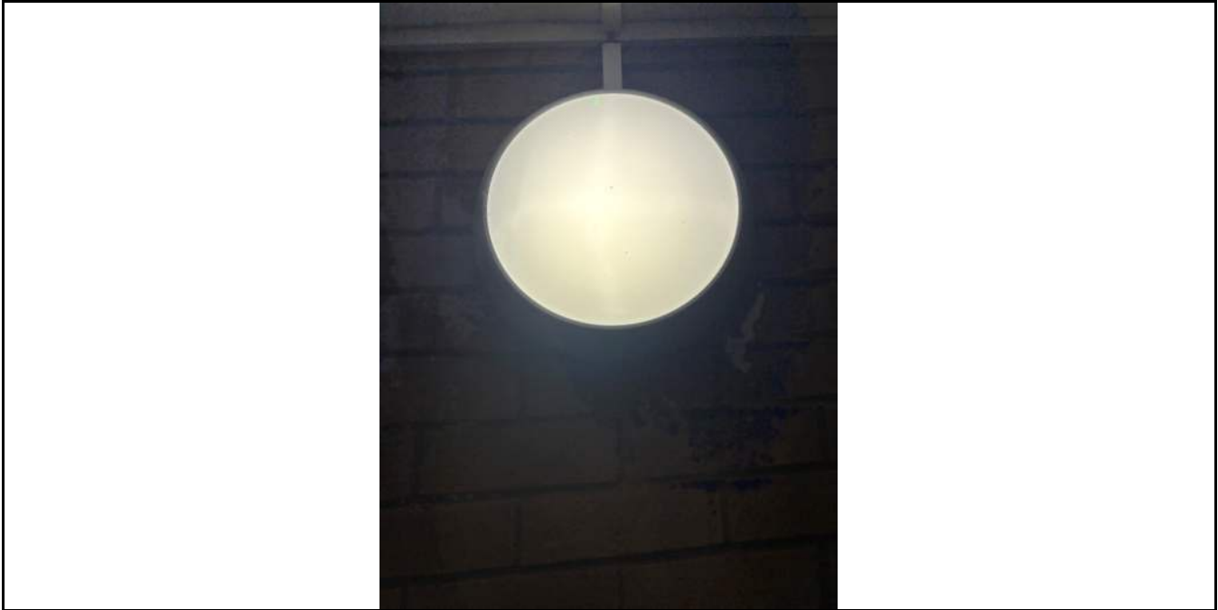
Photo No. 3 Emergency loighting in good condition and secured
