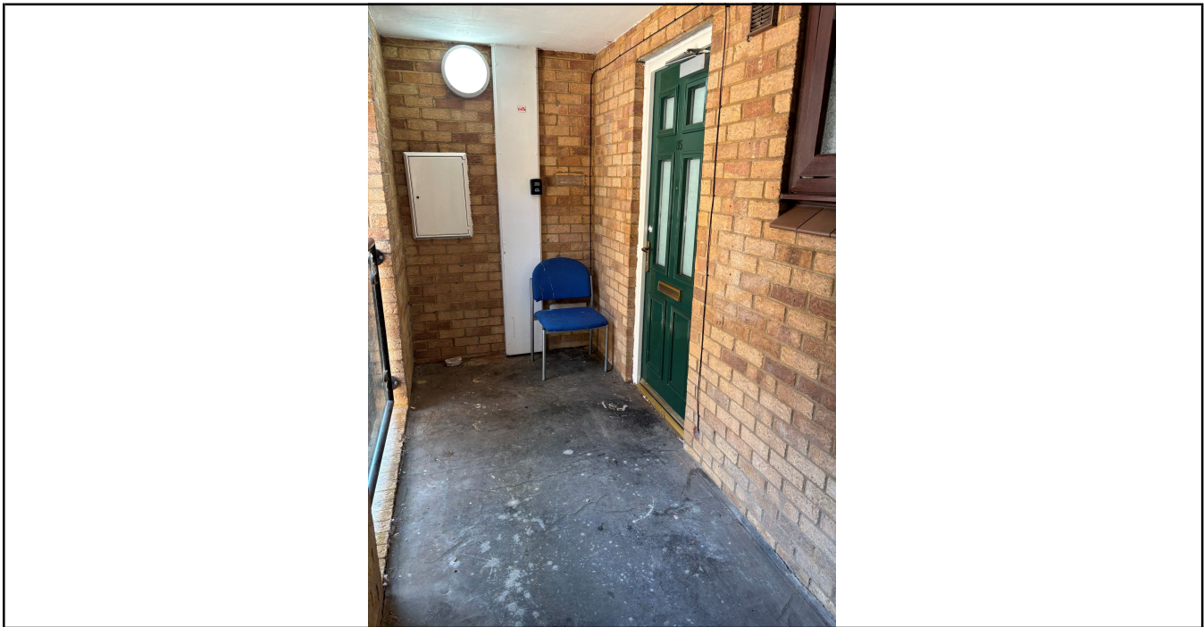
Photo No. 4 Personal items outside Flat 85
