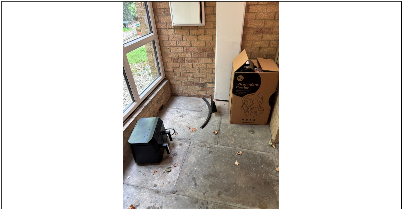
Photo No. 1 Personal items outside Flat 81
