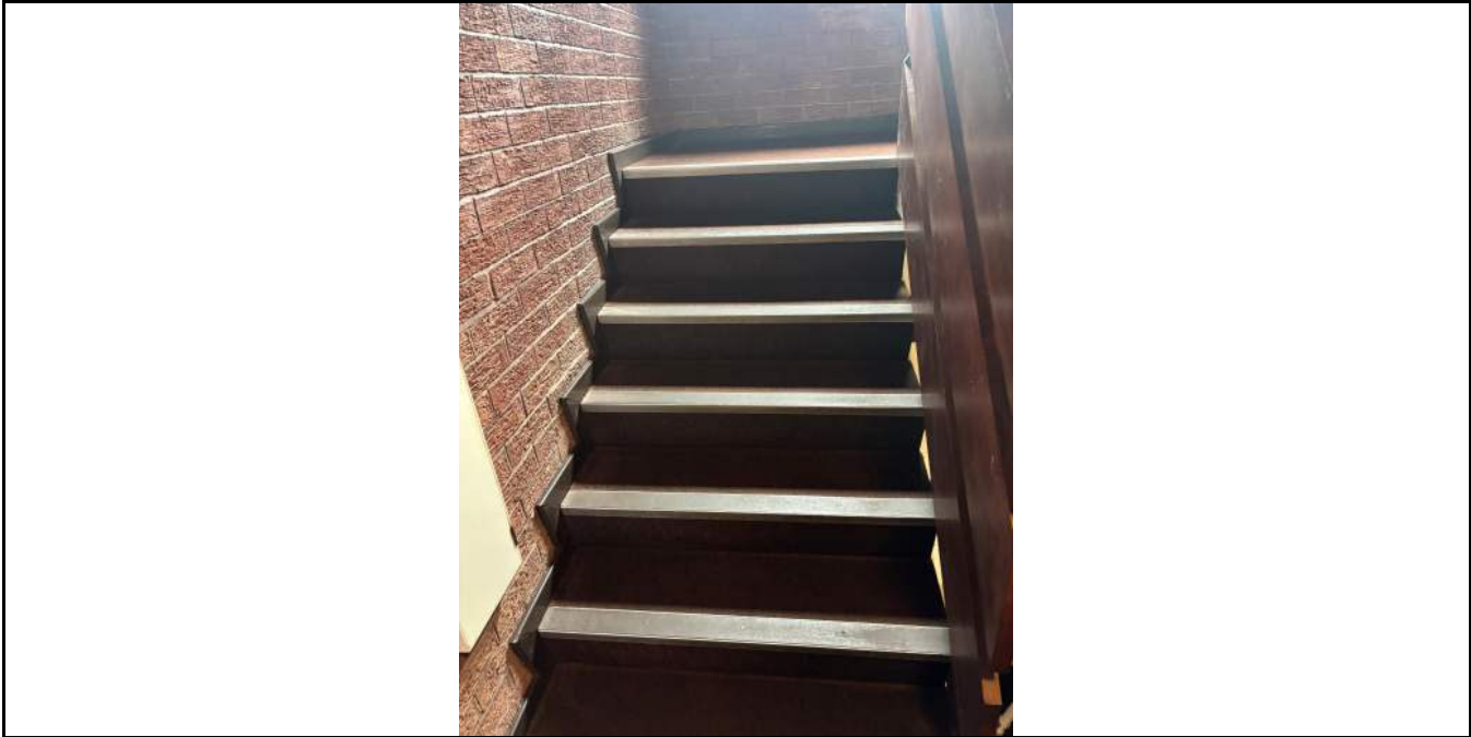
Photo No. 3 Clear means of escape
