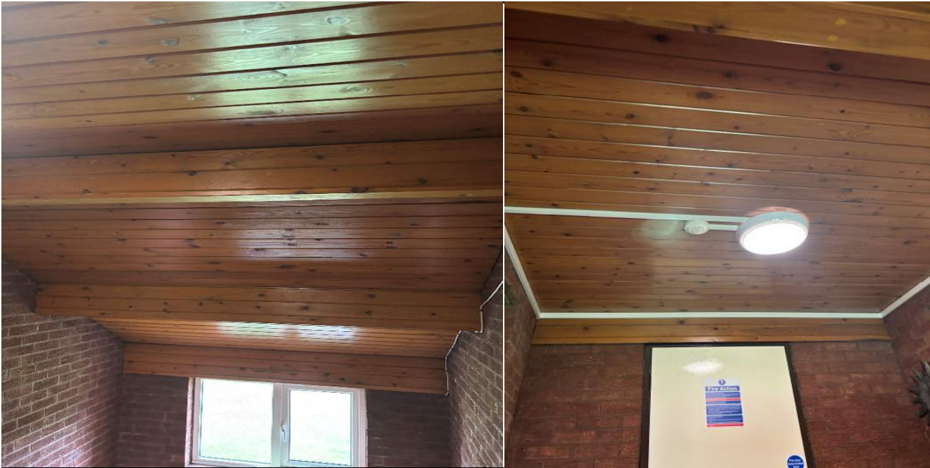
Photo No. 4 Timber cladding to ceiling on stairs and Landino 1st floor
