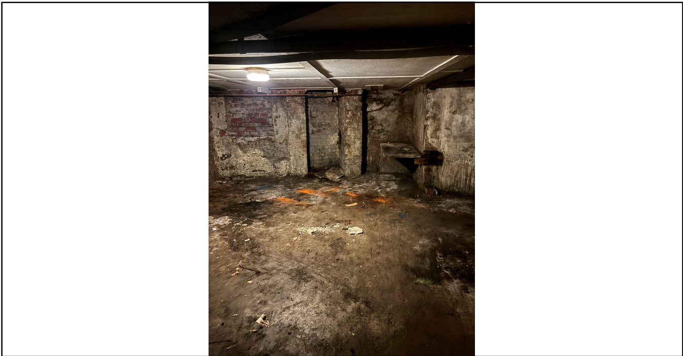
Photo No. 6 Basement clear of items
