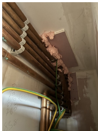
Excessive use of expanding foam.
