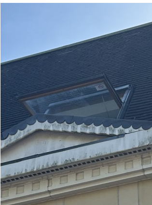
AOV in open position - external.
