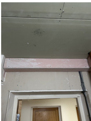
Non-fire -resisting plasterboard used in services cupboards.
