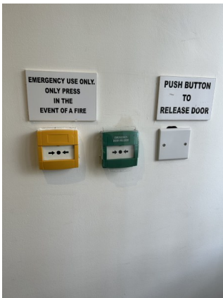
Example of control for door exit.
