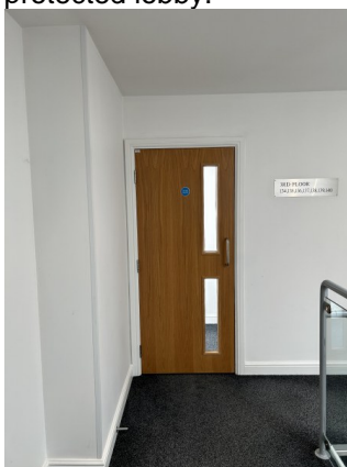
Example of fire door providing lobby protection.
