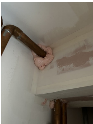
Excessive use of expanding foam.
