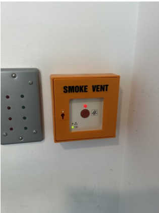
AOV control switch showing red fault light.
