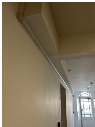
Example of wires liable to collapse.
