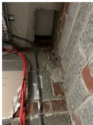
Lack of fire separation between floors.
