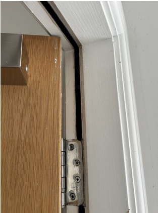
Common part fire door fitted with intumescent strips and cold smoke seals.
