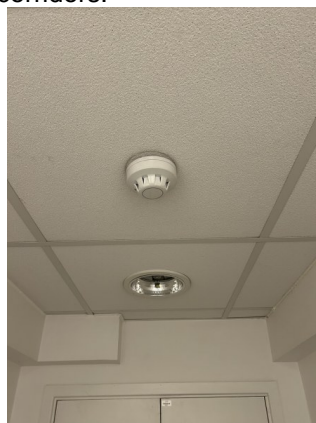
Example of smoke detection.
