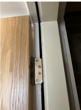
Services cupboard doors fitted with intumescent strips and cold smoke seals.
