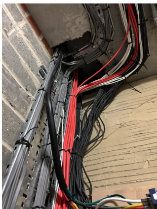
Lack of fire separation between floors.
