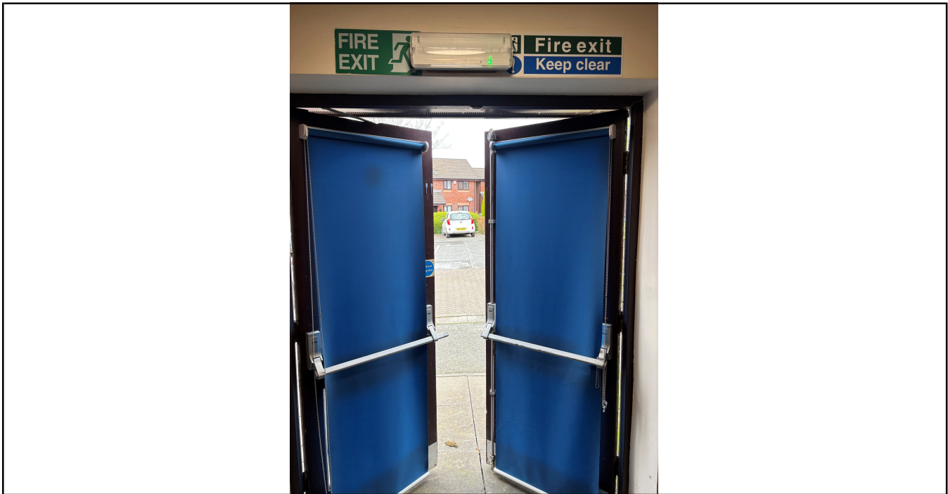
Photo No. 2 Escape doors open onto clear area.
