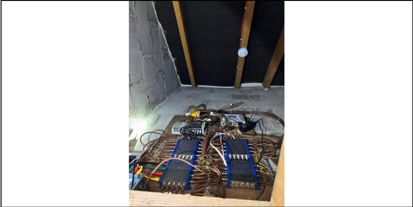
Photo No. 9 Detection in loft area
