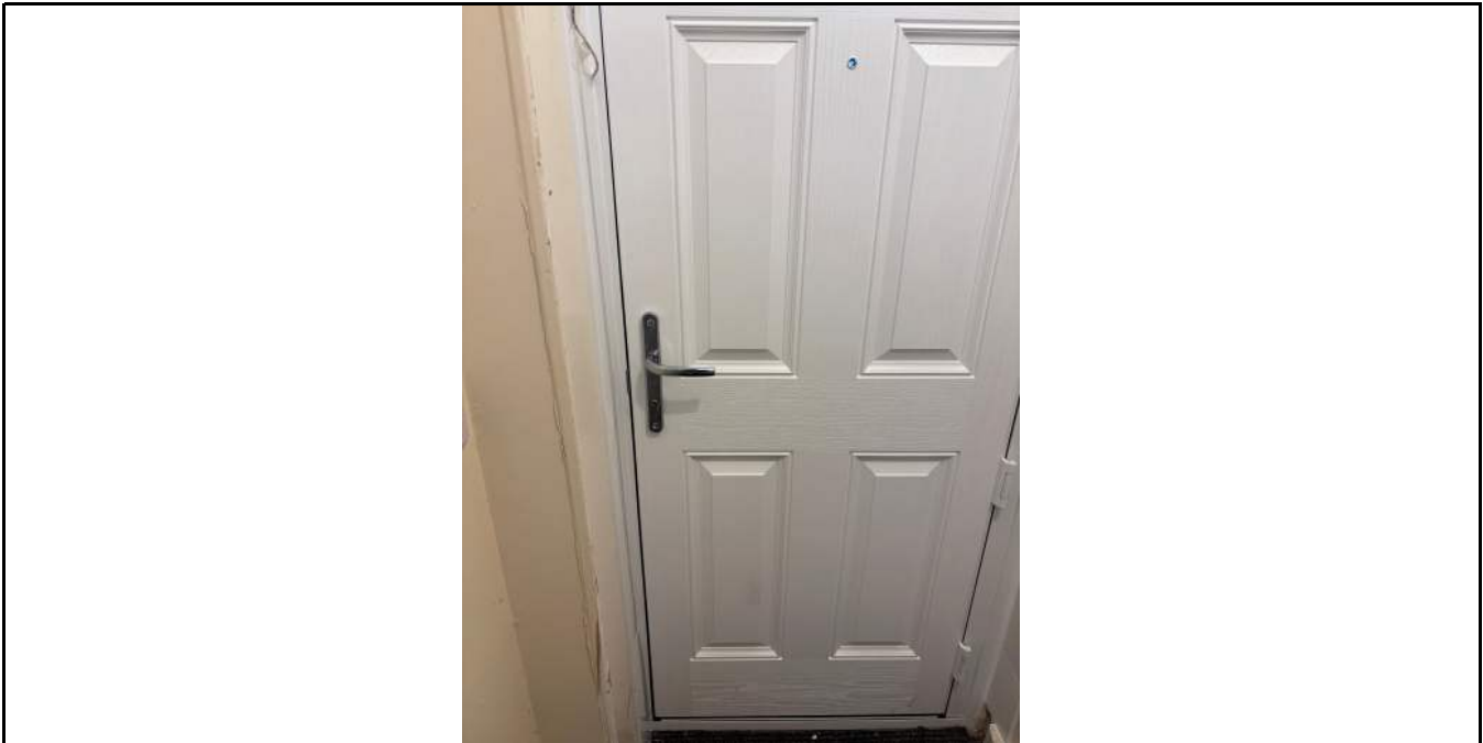
Photo No. 6 Main entrance door with key operated handle.
