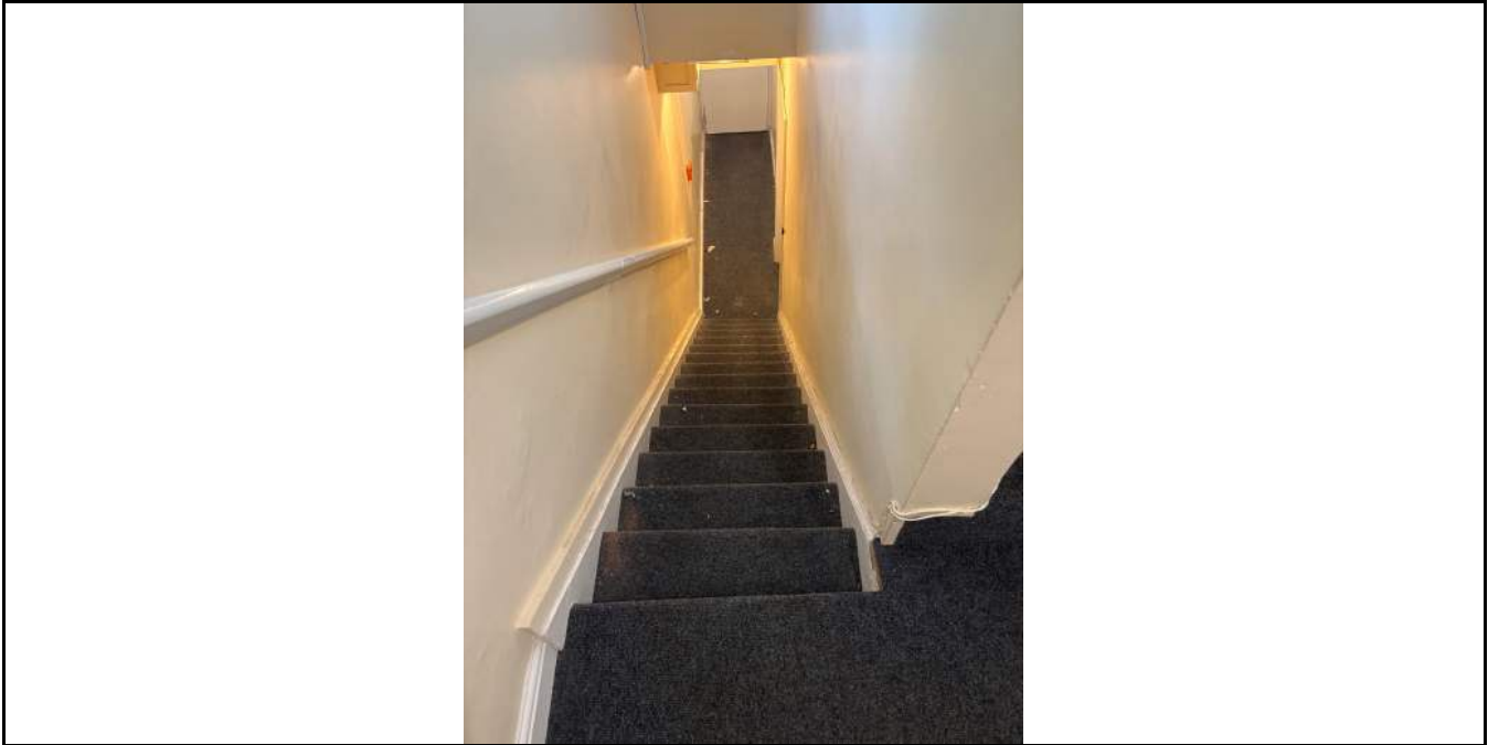
Photo No. 5 Clear means of escape
