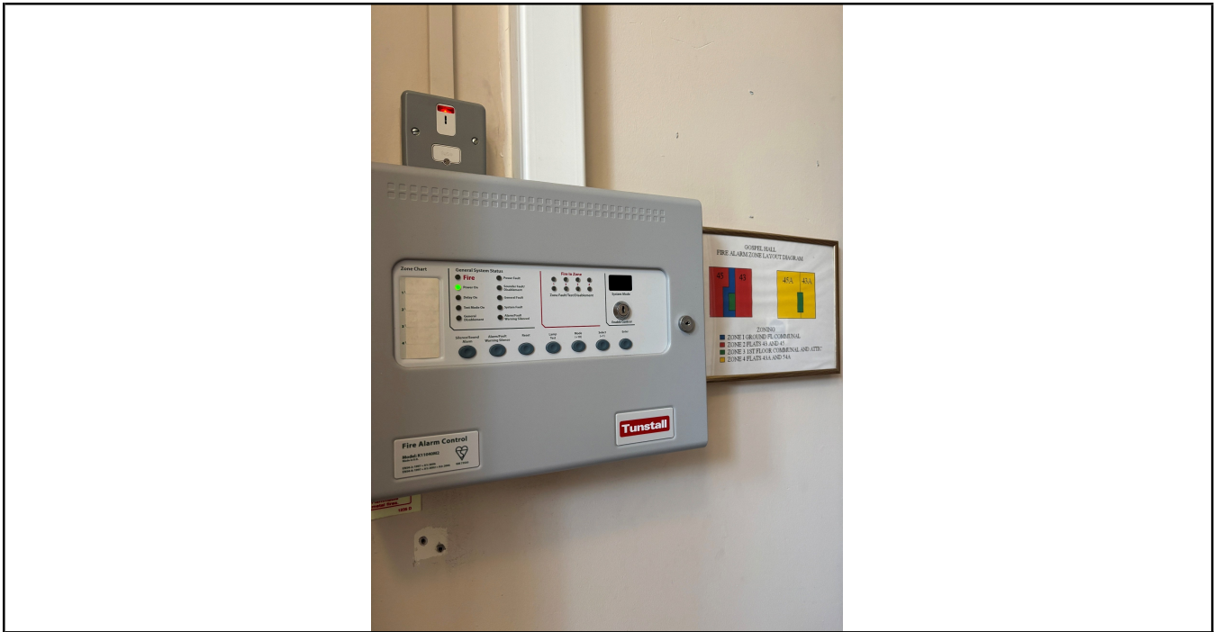
Photo No. 3 Fire panel healthy with zone plan
