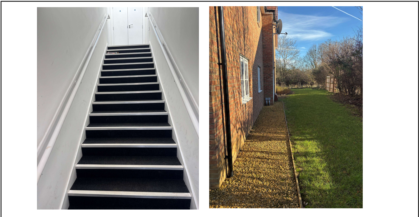
Photo No. 6 All escape routes were clear at the time of the audit.
