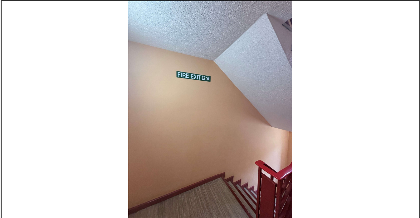
Photo No. 4 Exit Signage
