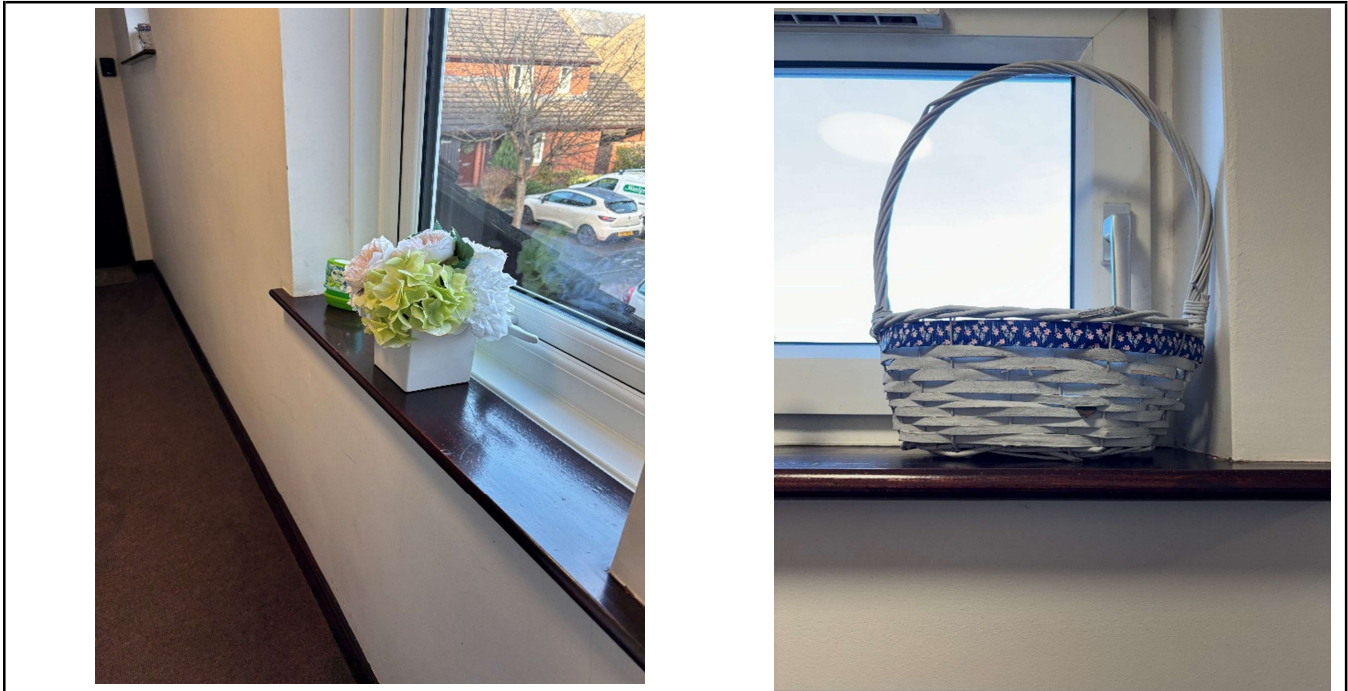
Photo No. 1 Combustible items in hallways
