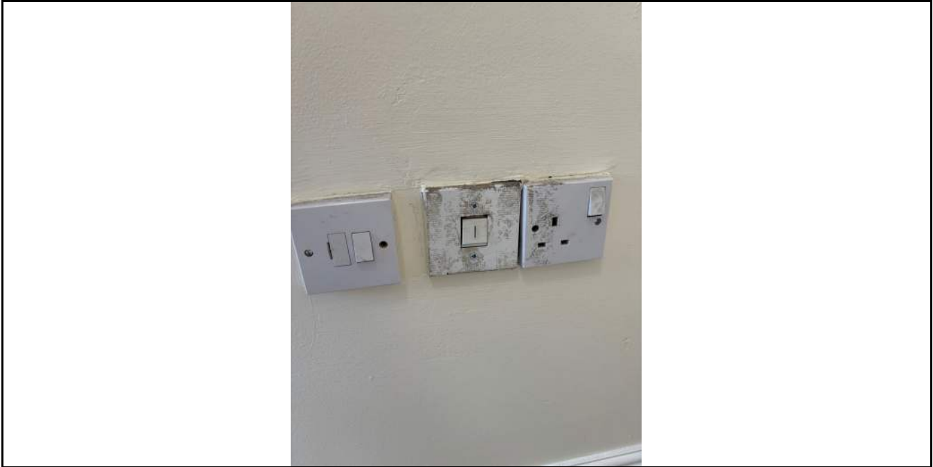
Photo No. 3 Electrical sockets in working condition
