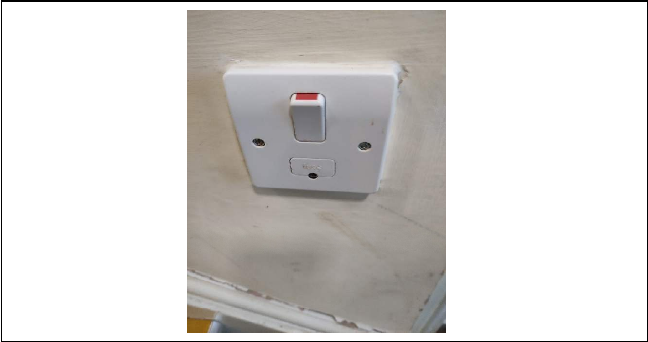
Photo No. 1 Sockets in good condition.
